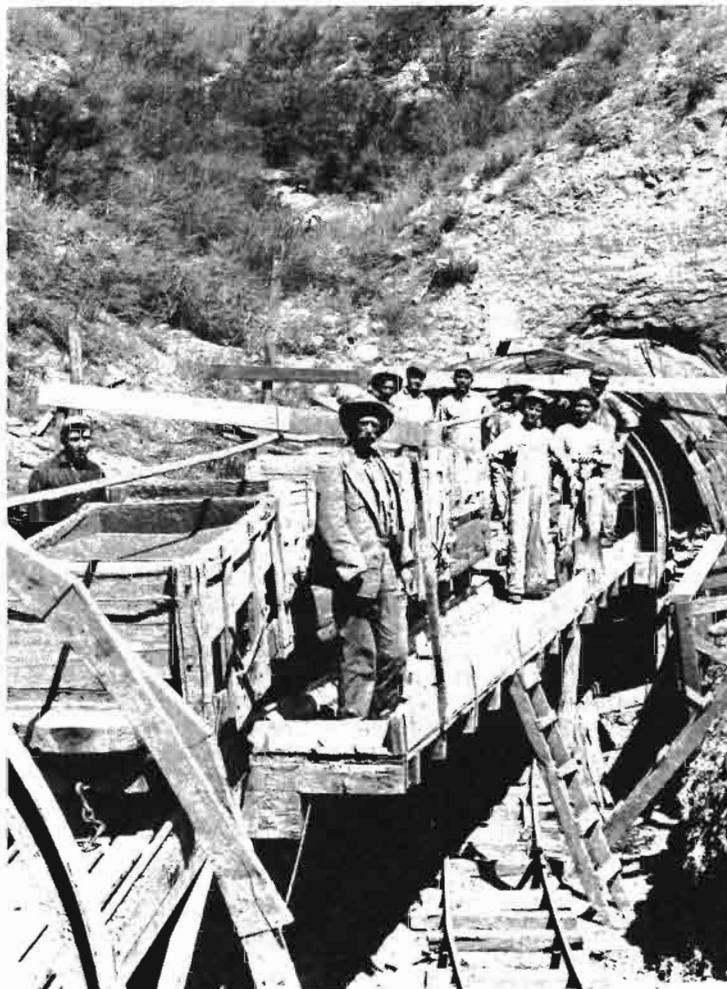
A scene from the construction of the Owens Valley Aqueduct, 1908. [Courtesy L.A. Department of Water and Power.]
